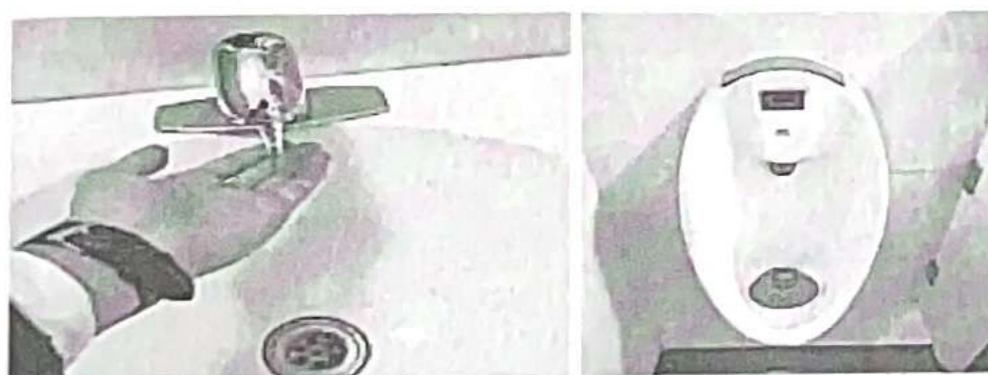
Fig. 3 - Sensor based hand wash taps and water less urinals.
