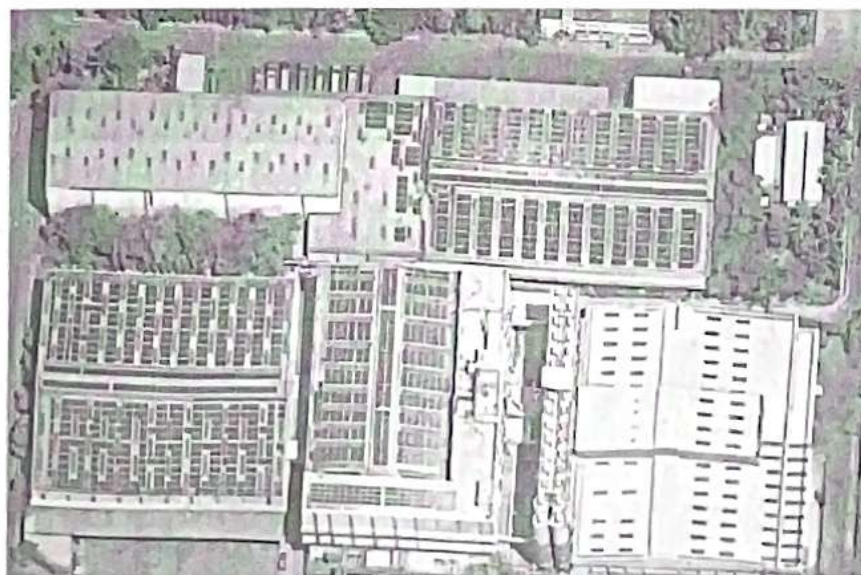
Fig.6 – Roof top solar inside the plant.
